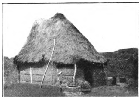
FIG. 5.—View of Exterior of Shed.
